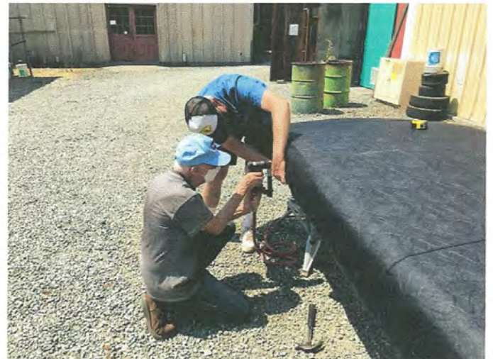
Stretching and Stapling Canopy Vinyl
