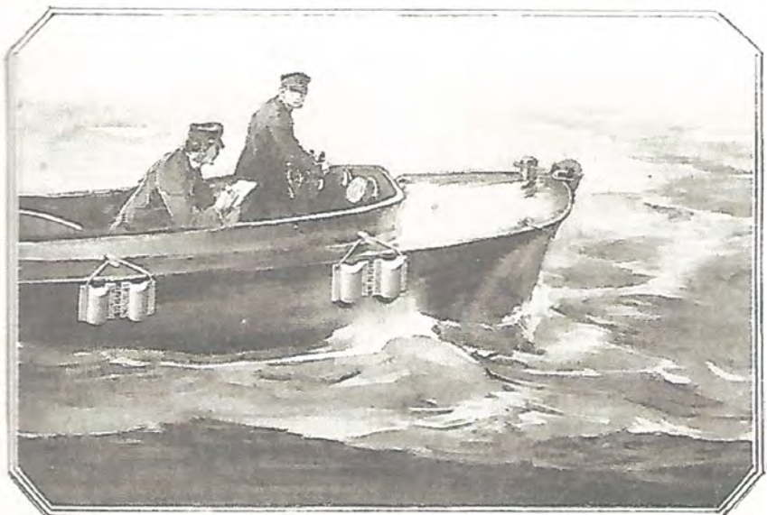
Having done their duty ashore, send 'em to sea. Cut into uniform sizes, laced and hung as illustrated, they make efficient buffers
