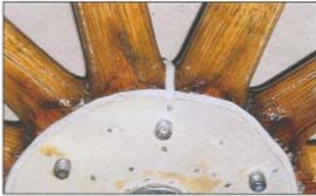
Sealing between spokes and Mortite sealer tips.
